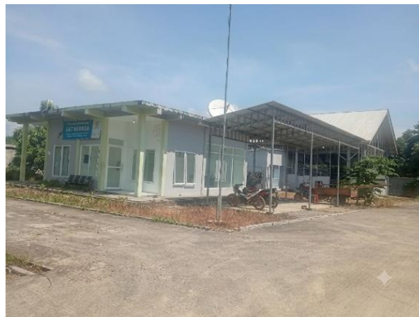
Figure 2. The condition of the location of PLTD is felt.
